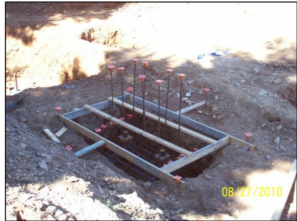
Figure 11: Dimensional Lumber Formwork at Top of Pile Cap
