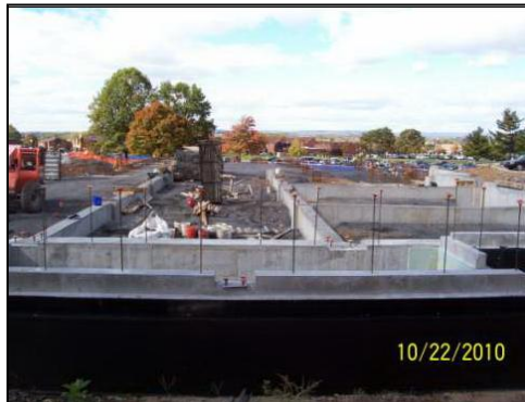
Figure 13: Grade Beams & Foundation Walls at East Side of Building
