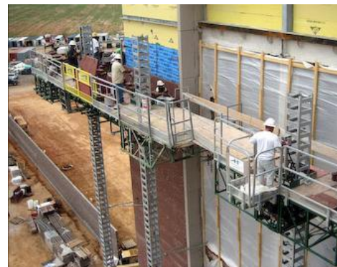
Figure 13: Typical Hydro-Mobile Scaffolding. Image taken from hydro-mobile.com
