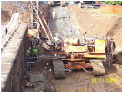
Figure 10: Steel Soldier Pile Installation at Existing Tunnel
